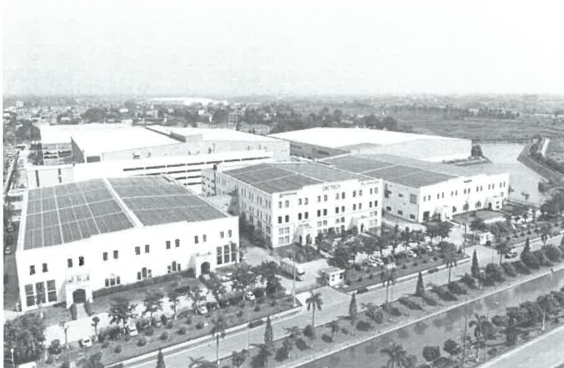
Figure 5: Image of CNCTech Thang Long factory in Phu Tho
